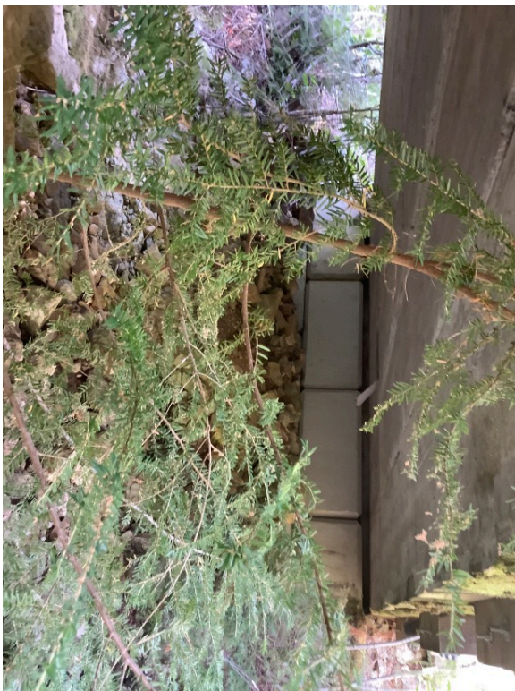
Right Bank Abutment when facing downstream
